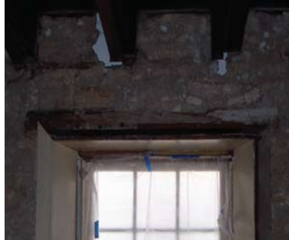
Angled Window Frames and Exposed Coquina Stone Why is the coquina exposed? Read the next article.
