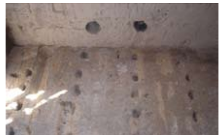
Shelving Holes in Coquina Wall
