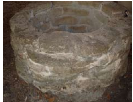
Coquina Well with Quicklime Mortar
