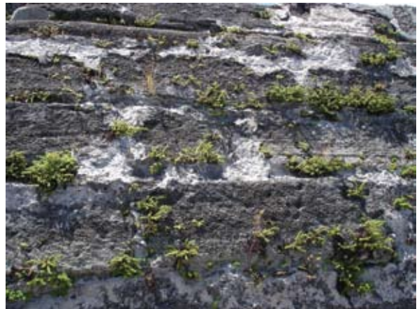
This is a close-up of a coquina well at the Turnbull foundation. Many plants are growing right on the coquina blocks.
