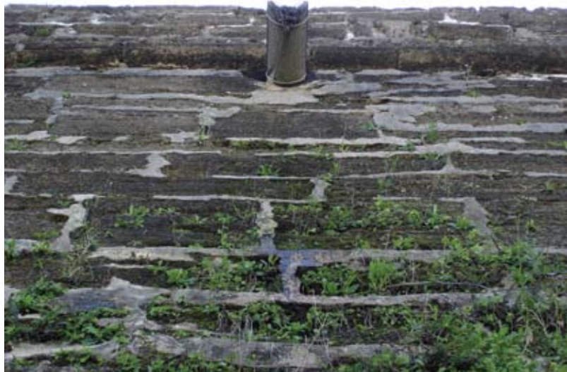
Image 2: View of Castillo Scupper
