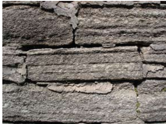
Repointed Coquina Wall
