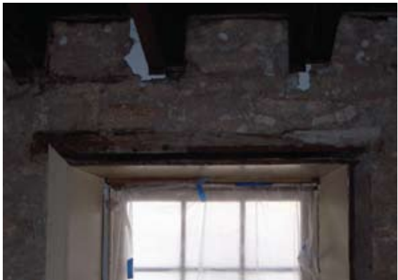
Portland Cement Fix at Ximenez-Fatio House
