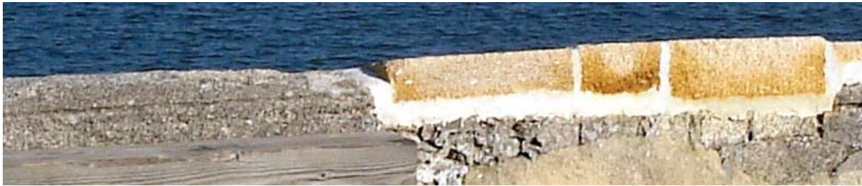
Conservation Work Showing New Coquina Blocks Added at the Castillo
